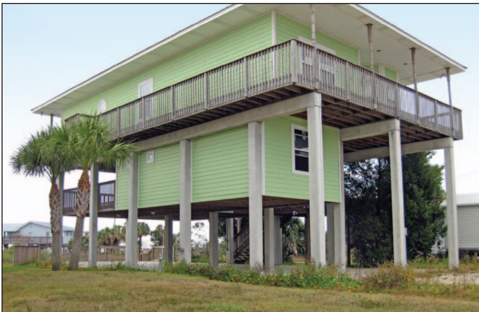
Figure 2-23. Above-grade enclosure (Perry, FL)
